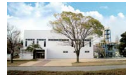
Outside the Operation Training Center
