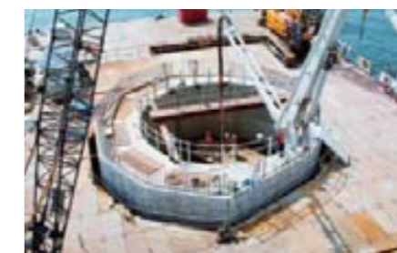
CelcreteH® used in underwater concrete placement activities
