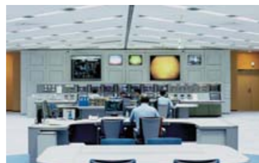
Operations room of the integrated production center at Aboshi Plant
